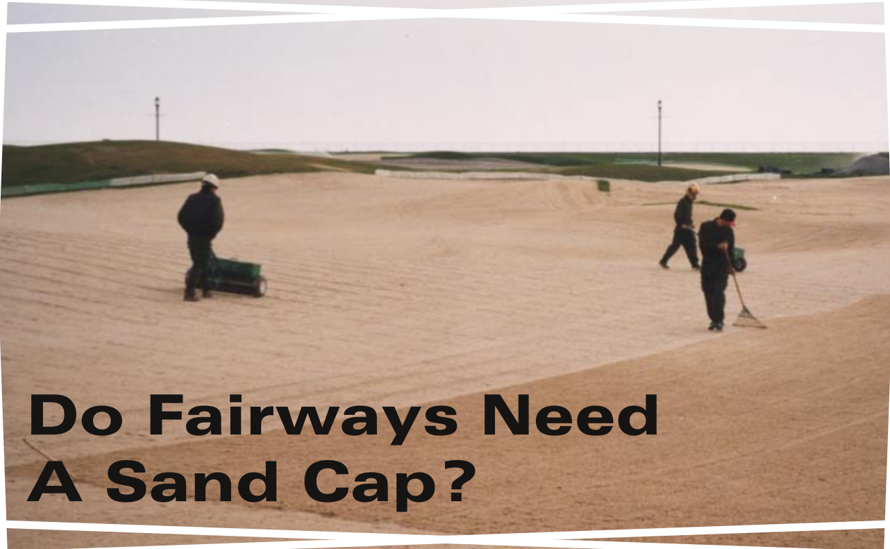
Fig.1: Spreading seed on a sandcapped fairway at Shanghai.
